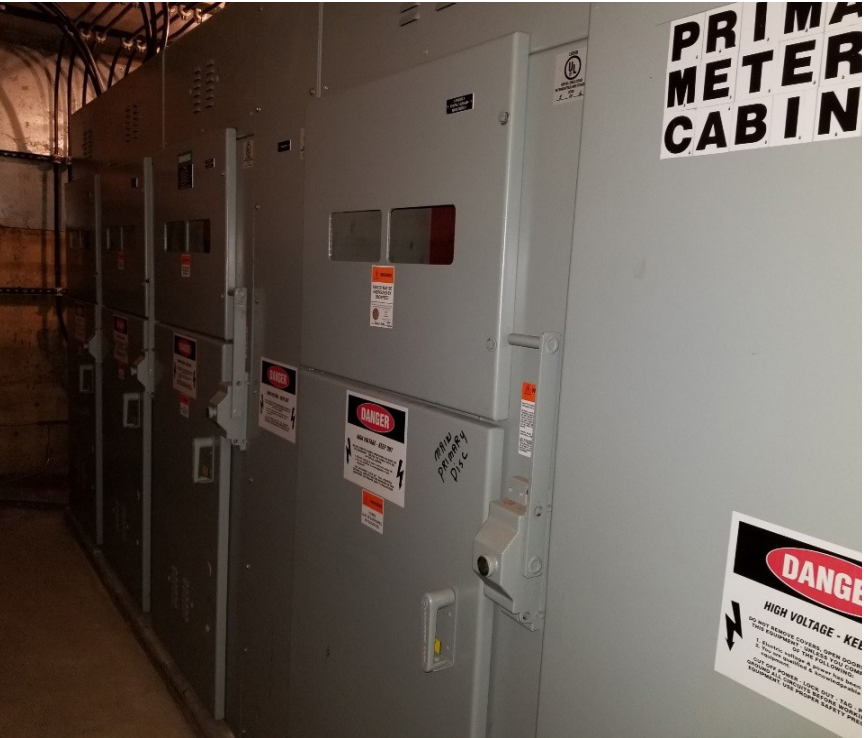
ComEd Vault Switchgear
