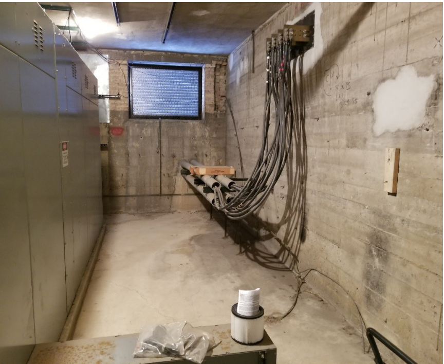
Secondary Cables to Basement Electrical Room
