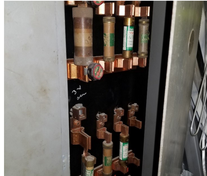
Live-front Distribution Equipment – Basement
