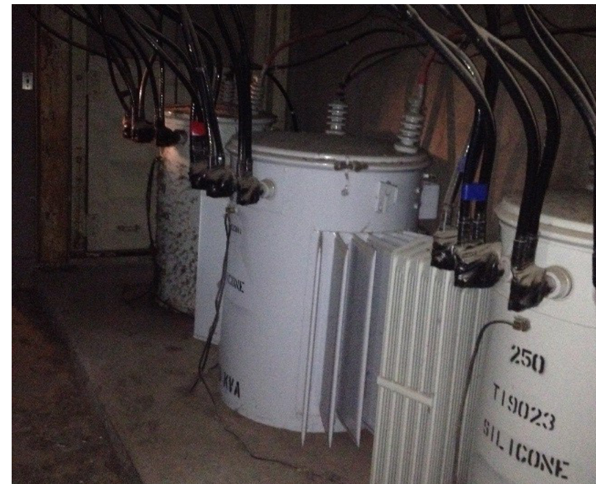
Indoor Transformers Feeding First Floor Electrical Room
