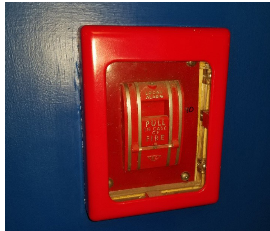
Fire Alarm Pull StationElectrical Room
