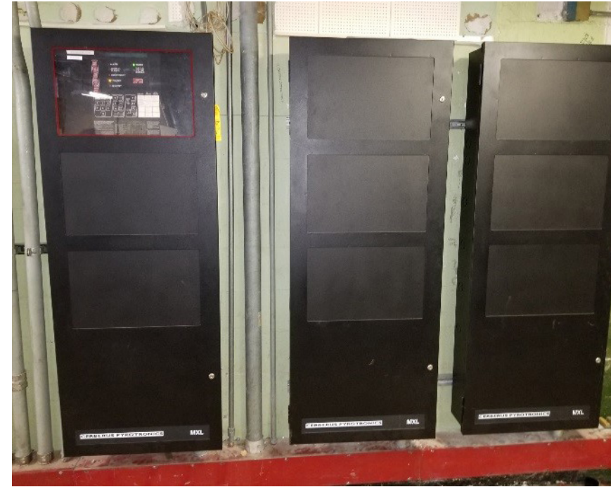
Fire Alarm Control Panel
