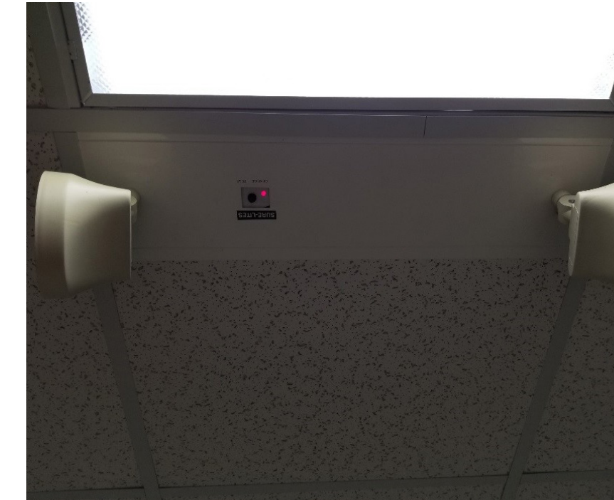
Emergency Lighting – Ceiling Mounted
