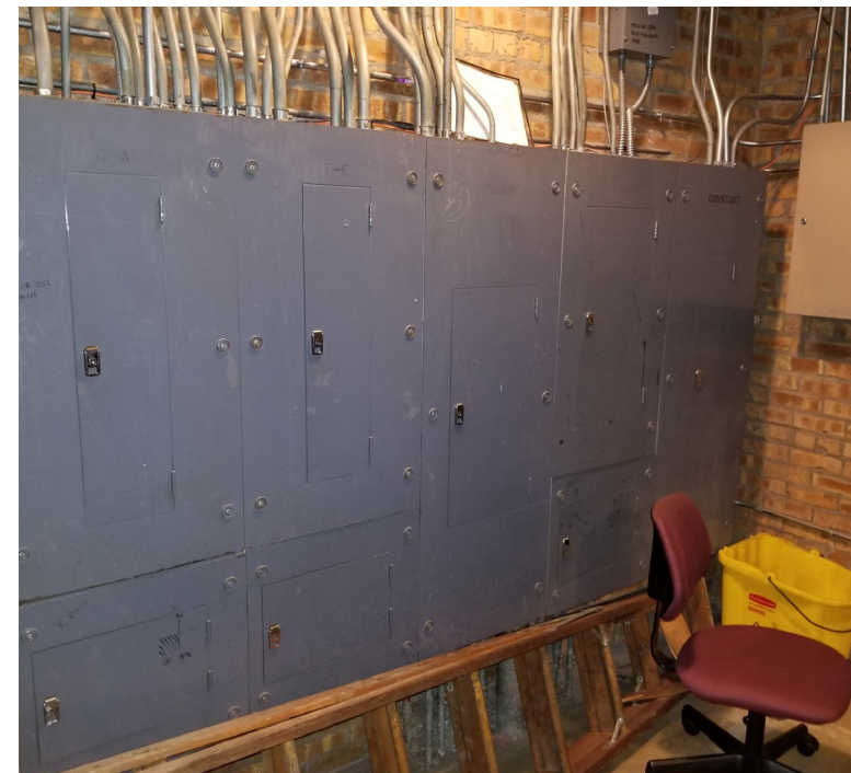
Substation C-1 Distribution Panels
