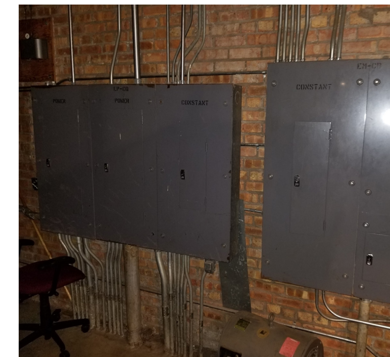
Substation C-2 Distribution Panels
