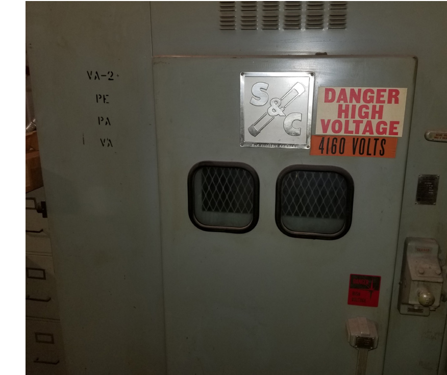
Substation VA-2 4160V Switch
