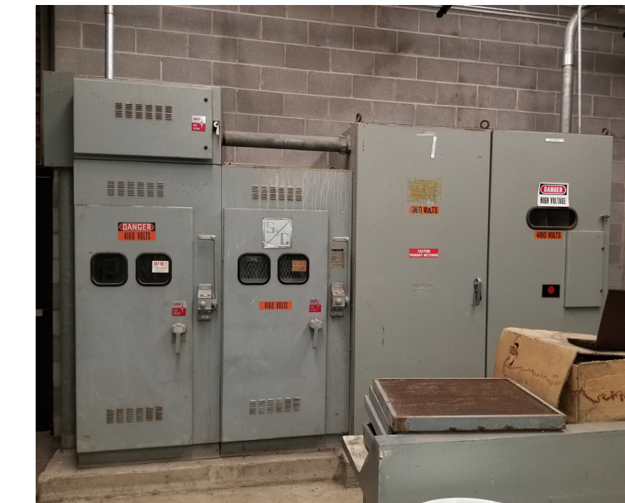
Cogeneration Building 4160V Switches
