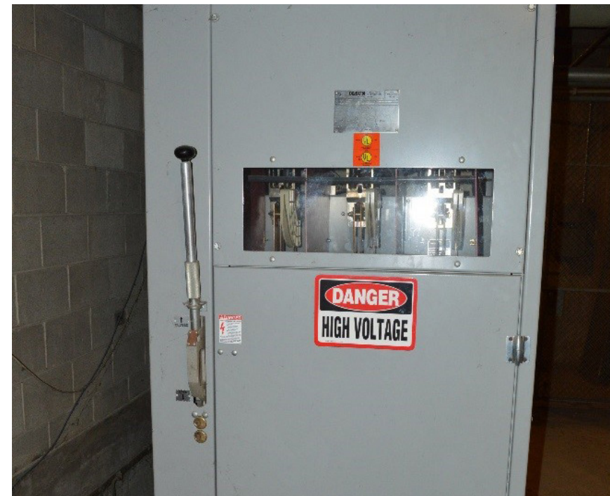
B-Wing Substation Load Break Switch
