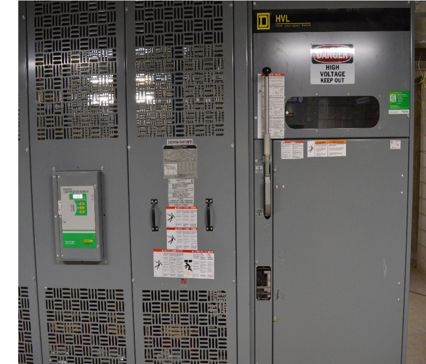
E-Wing Substation #2 – Load Break Switch and Transformer
