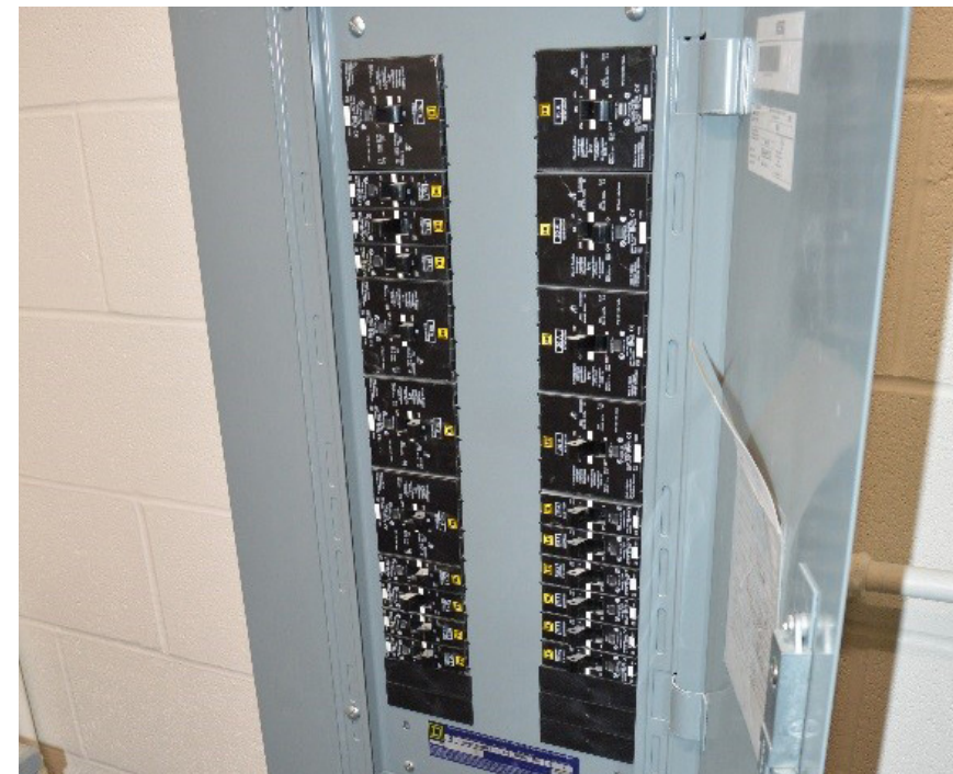
New 480V Panel – From E-Wing Substation #2
