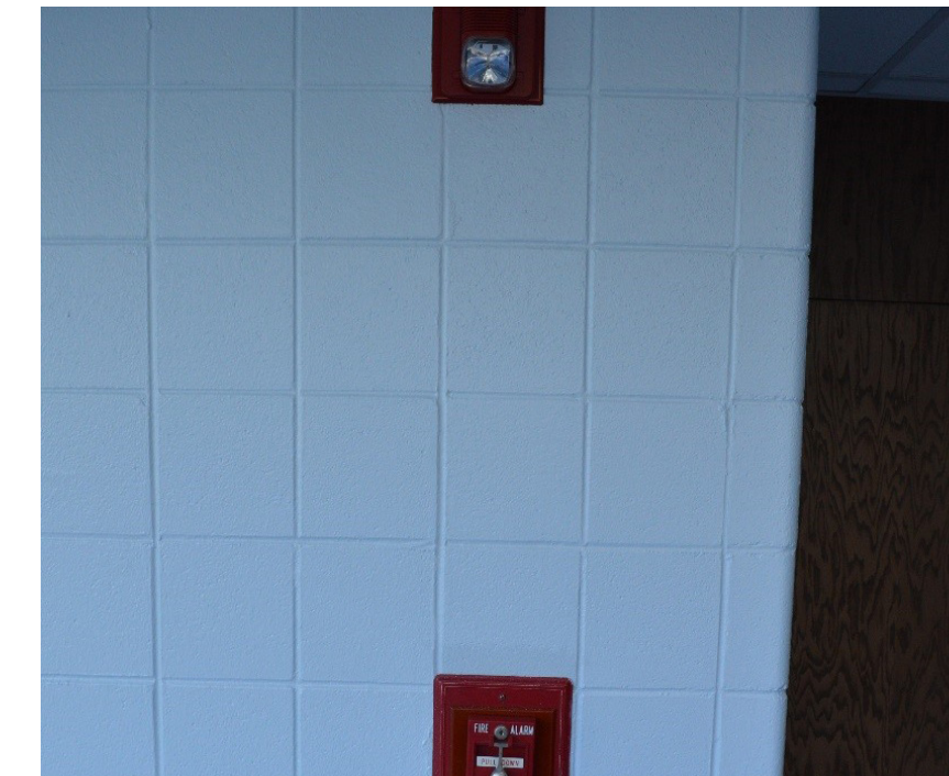
Fire Alarm Pull Station and Visual Device
