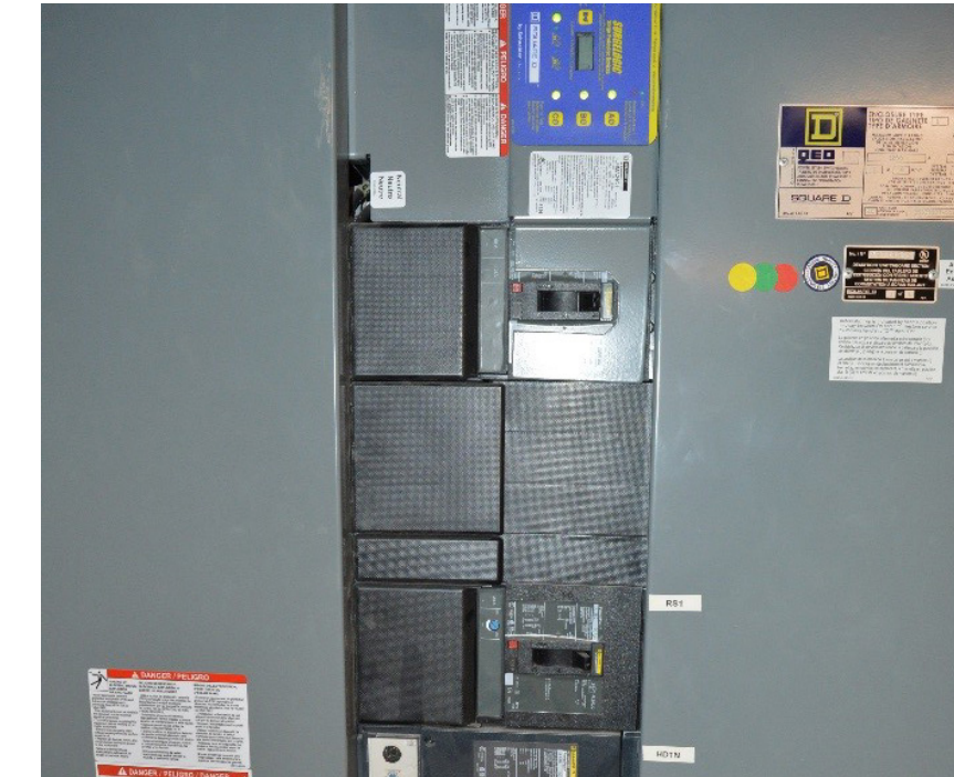
E-Wing Substation #2 Branch Circuit Breakers
