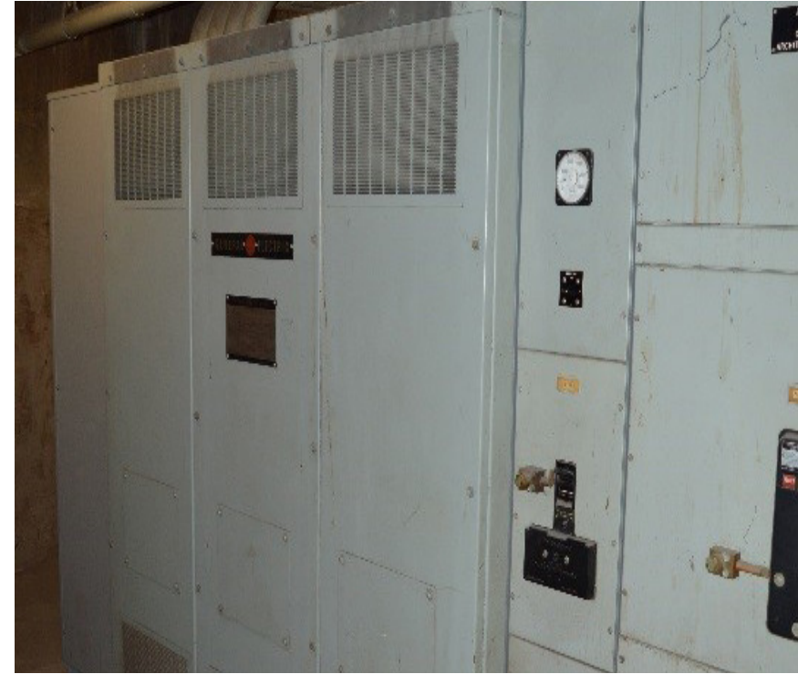
Center Core Substation – Transformer and EM Breaker
