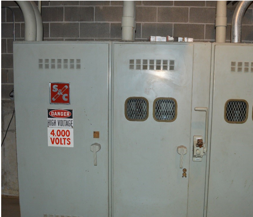
B-Wing Substation 4160V Switch
