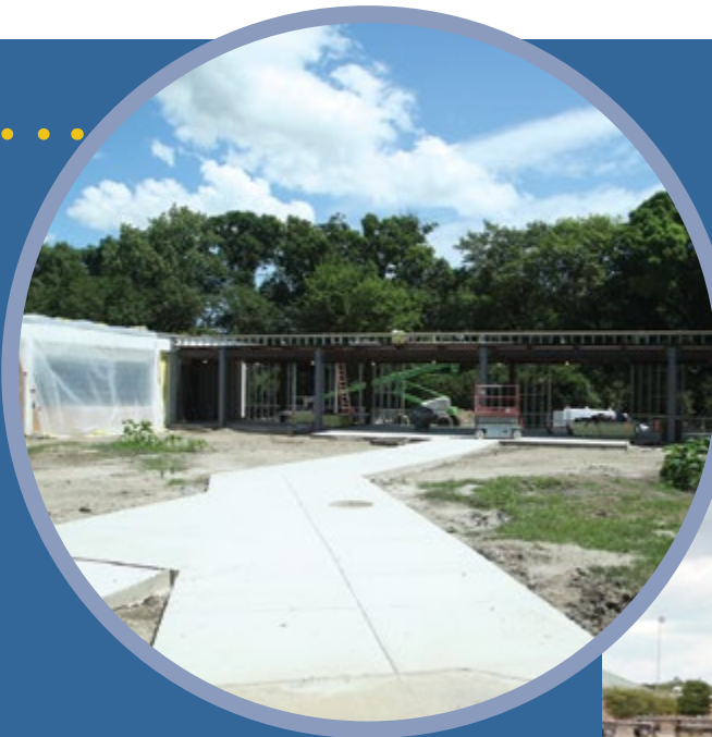
The construction of a new hallway that will connect the main building at Maine South with A wing is in progress.
