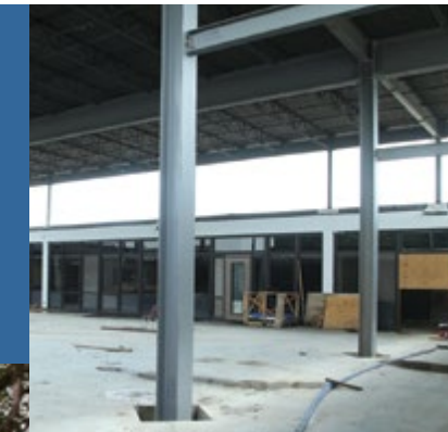
With steel supports installed, work begins on transforming the former courtyard into space for the new cafeteria at Maine South.
