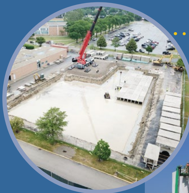
An aerial view of the retention vaults installed at Maine West.
