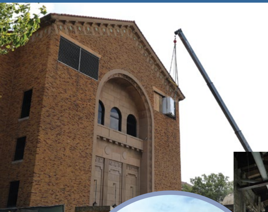
Materials are delivered by crane to the third floor of Maine East as that floor is converted into fine arts space.
