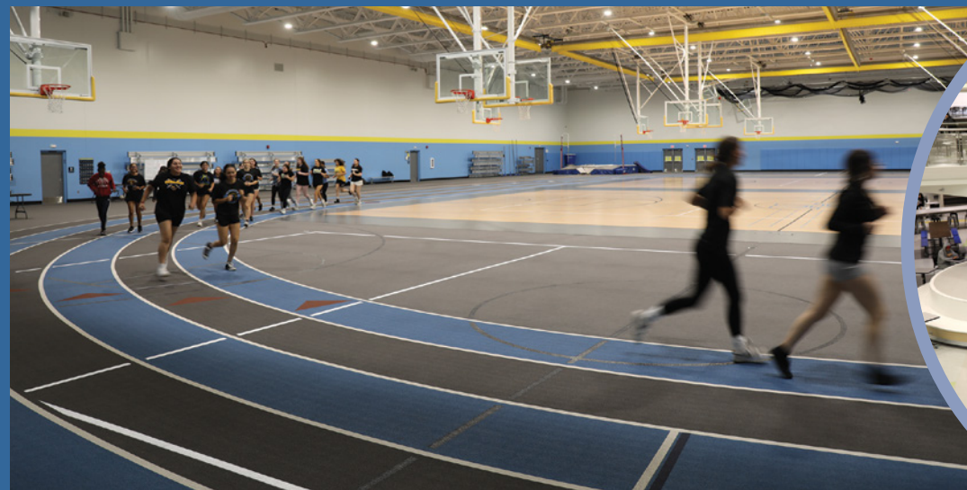
The new fieldhouse (right) at Maine West is a completely new structure that is utilized for physical education classes and competitions.
