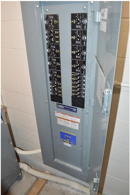
New 480V Panel – From E-Wing Substation #2 (Spectator Gym)
