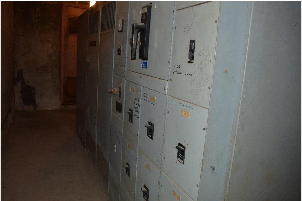
A-Wing Tennis Court Lights Transformer Load Break Switch
