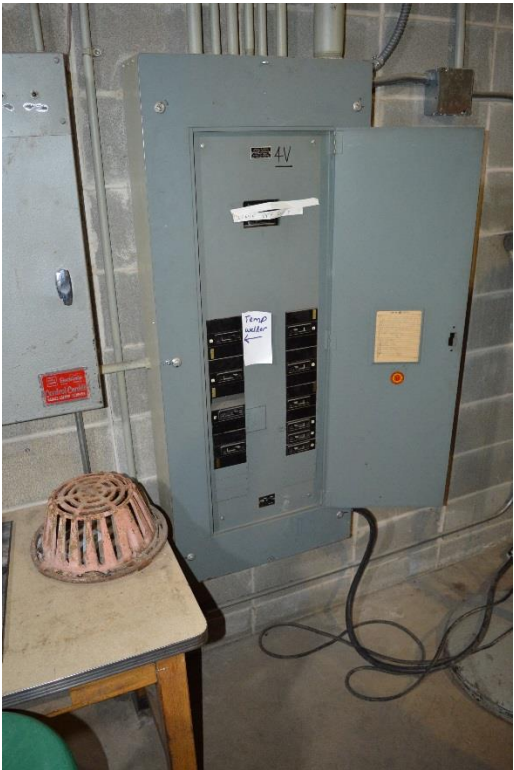
New 480V Panel – From E-Wing Substation #2 (Spectator Gym)
