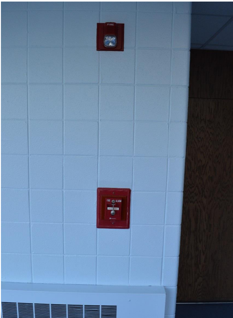
Fire Alarm Pull Station and Visual Device
