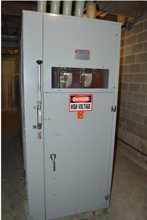
C-Wing Substation 4160V Load Break Switch
