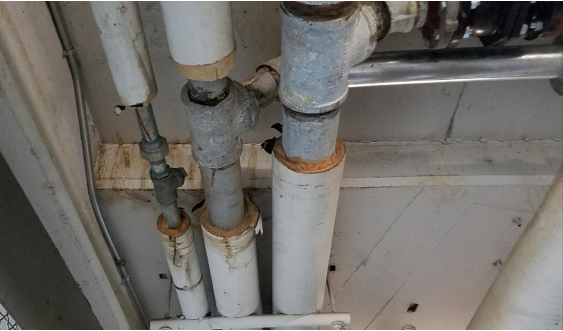
Sample of Existing Galvanized Piping
