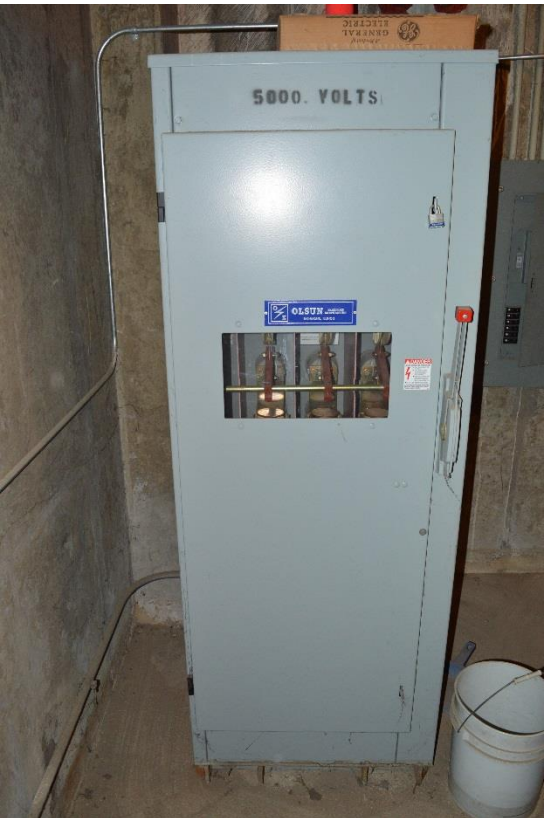
A-Wing Tennis Court Lights Transformer Load Break Switch
