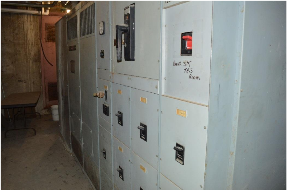
C-Wing Substation 4160V Load Break Switch
